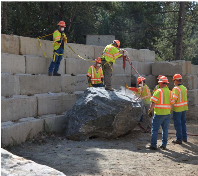
Figure 5. CDOT students drill into a rock during the Rock Fragmentation Training Course at the ERL.
