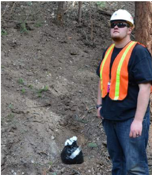
David Harper stands next to a carefully positioned case charge.
